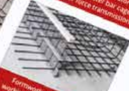
Formwork elements for working joints Stremaforme with coated metal water stop
