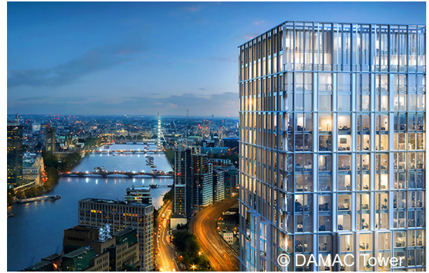
Nine Elms redevelopment, London Products: Shearail®
