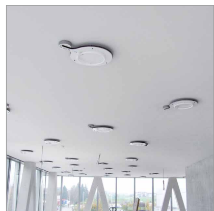
Surface appearance with acoustic plaster
