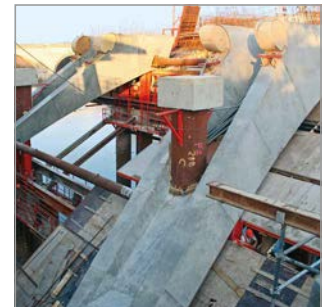
Grignac Bridge (FR), 2007
