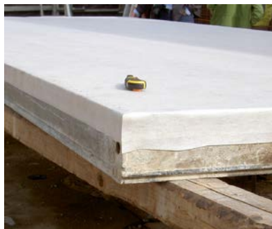
Formwork-liner self-adhesive fixed to the formwork
