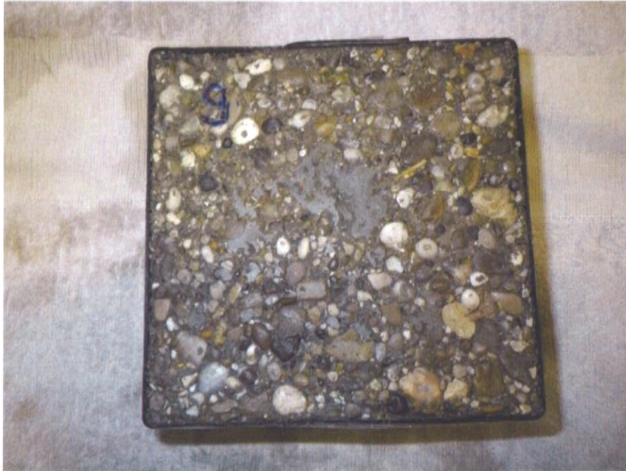
Picture 8: Sample 9 after 28 freeze thaw resistance, abgewitterte surface. No damage on the spacer recognizable.
