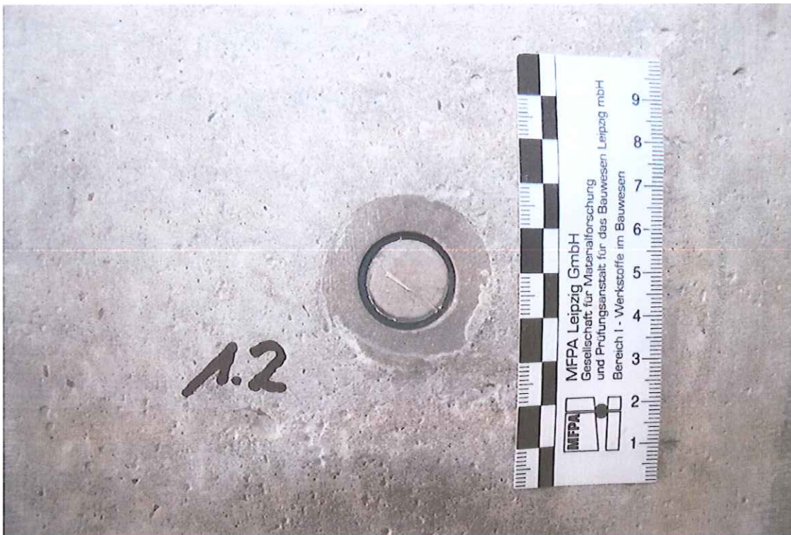
Figure 2: The sealing plug of test specimen 1.2 after the pressure test
