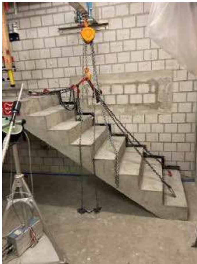
Figure 41: Installation situation stair flight
