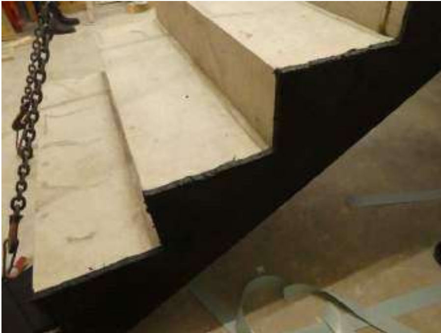
Figure 18: Stair flight with distance plate FDPL 15420 during installation
