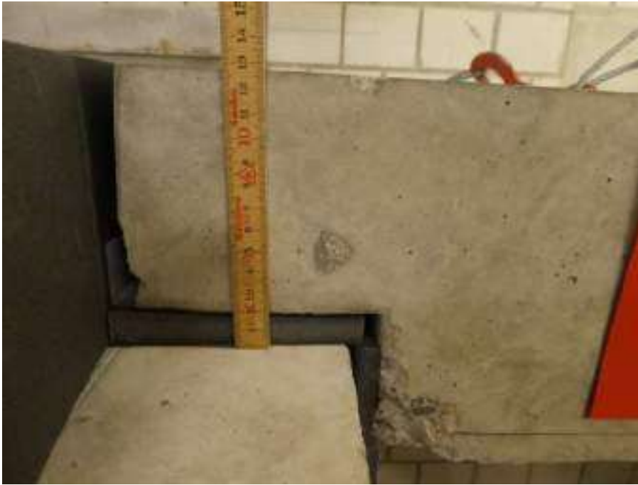
Figure 16: Staircase bearing Egcoscal SP LS 43 kN in installed state (top)
