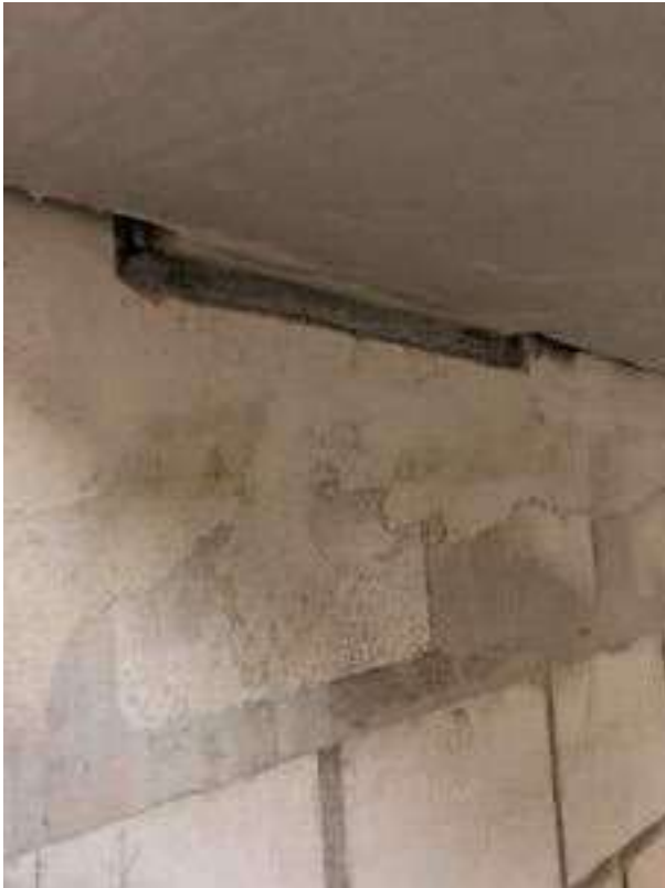
Figure 20: Stair landing bearing Egcosono SP with 15 mm elastomer bearing after finished installation, z = 1.5 cm
