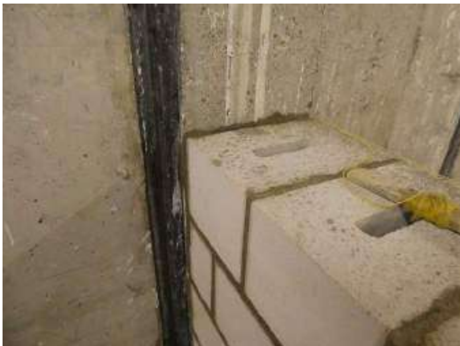
Figure 25: Detail of the masonry
