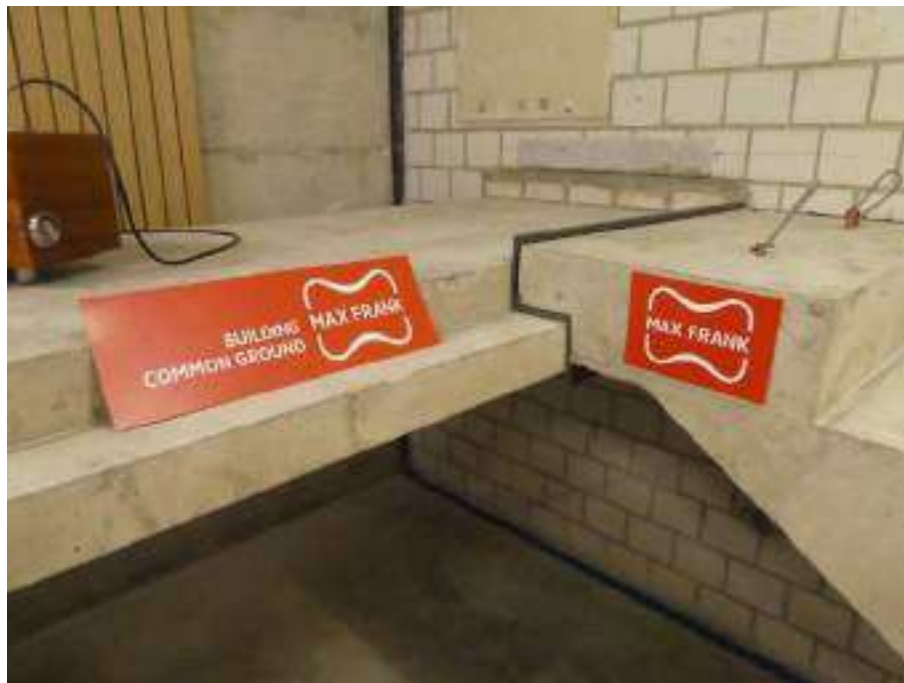
Figure 39: Overview of installation situation – measurement of stair flight impact sound pressure level
