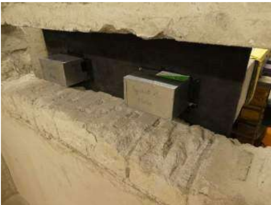
Figure 21: Stair landing bearing Egcopal SPX with 15 mm elastomer bearing during installation
