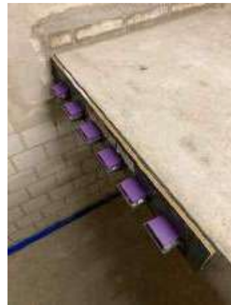
Figure 4: Detailed view of Egcostep SP staircase bearing with 15 mm elastomer bearing, type S6 version
