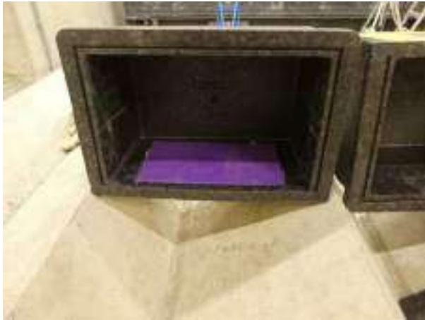
Figure 7: Stair landing bearing Egcosono SP with 15 mm elastomer bearing
