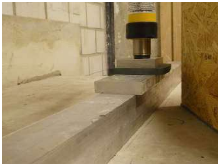
Figure 38: Applying the additional load on the stair landing (configuration 2)
