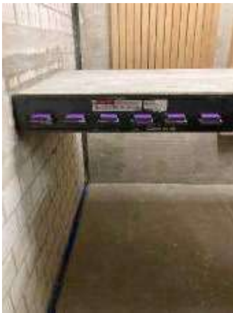
Figure 3: Staircase bearing Egcostep SP with 15 mm elastomer bearing, type S6 version, bearing at the top
