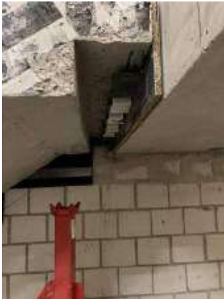
Figure 6 Staircase bearing Egcostep SP with 15 mm elastomer bearing, type S4 version, bearing at the top
