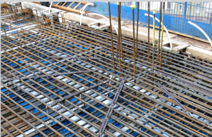
Figure 5 Placement of studs
